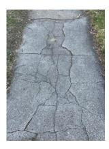
This is a picture of a broken sidewalk in our neighborhood. The cracks and holes make it hard for people to walk, especially for kids, older people, and those using wheelchairs or strollers. Fixing the sidewalk would make it safer and easier for everyone to get around.
